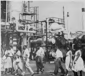
WALK, WALK is the way to see the plant, as tour groups find out. Actually there is a bus to take them around, but there's plenty of walking too, in places where buses can't go.
